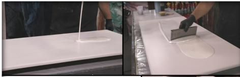
Pour the white epoxy out in the center of the project. Use a 1/8" notch trowel to spread the epoxy evenly
